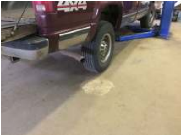
Photograph 17. View of sealed floor drain centrally located in main garage area within barn building – View to south.
